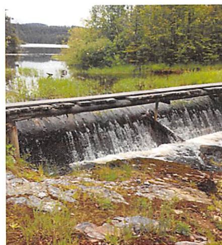
Oyama Lake Dam Spillway
