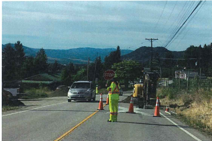
Water operators working along Okanagan Centre Road East
