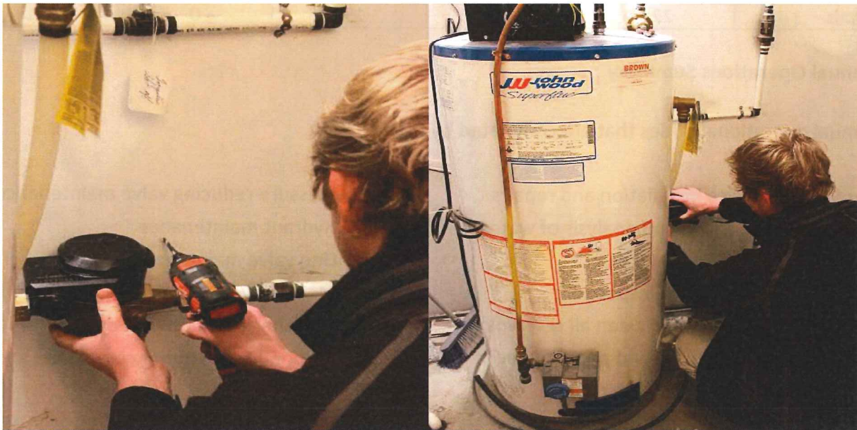
Neptune Meter contractor installing residential indoor meter (2015)
