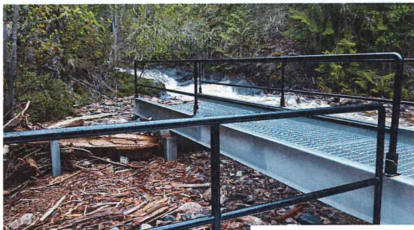
Oyama Creek Intake filled with debris.
