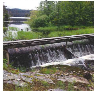
Oyama Lake Dam Spillway
