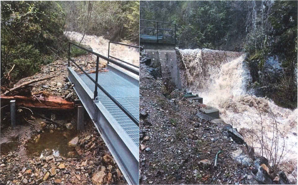
Left: Oyama Creek intake filled with debris. Right: High flows spilling over Oyama Creek intake.
