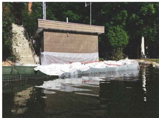
Lake Pine pumphouse
