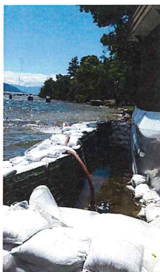
Lake Pine (left) and Coral Beach (right) pump-houses flood/high water protection measures.
