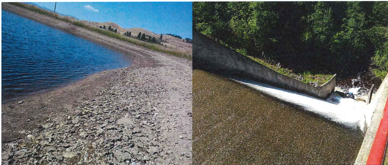
Eldorado drinking water reservoir (left) fed by Vernon Creek Intake (right).
