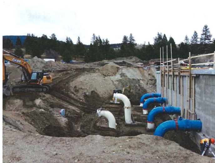
Treated reservoir construction at Eldorado
