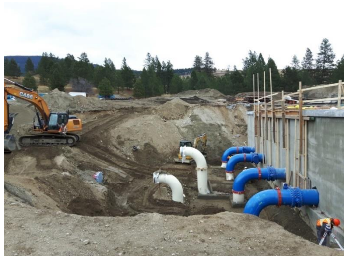
Piping being installed to new Treated Water Reservoir
