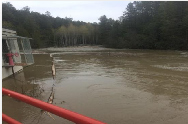
2017 Flooding of the Vernon Creek Intake Pond
