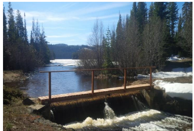
Right: Oyama Lake dam spillway.
