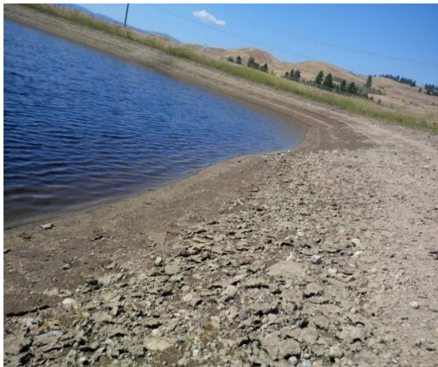
Left: Eldorado drinking water reservoir
