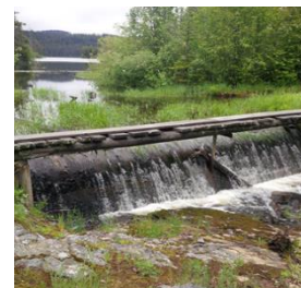
Oyama Lake Dam Spillway
