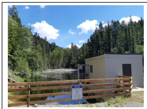
Vernon Creek Intake
