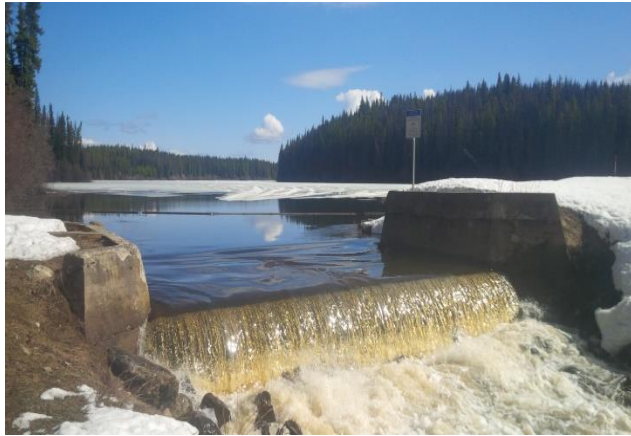
Left: Crooked Lake dam spillway
