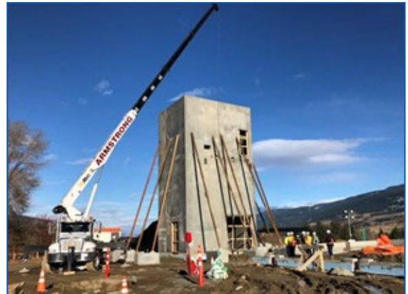
New Firehall under construction on Jardines Road
