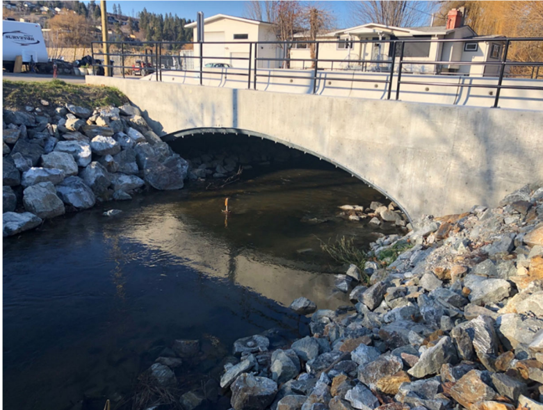
Figure 3. Reimche Road creek crossing installed during 2018
