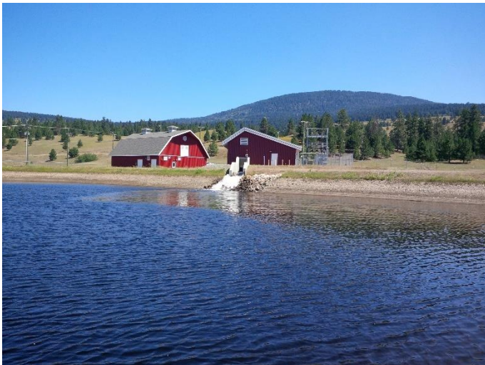
Left: Eldorado drinking water reservoir
