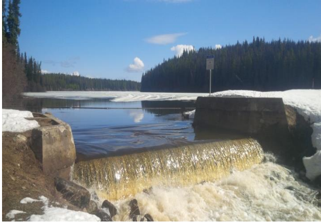
Left: Crooked Lake dam spillway
