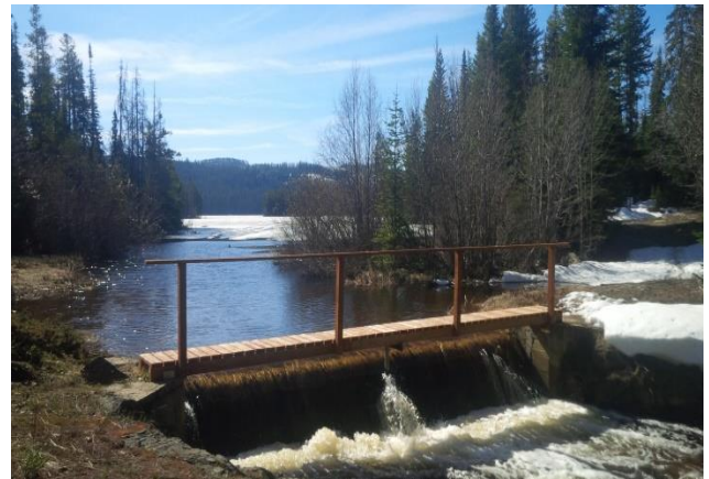
Right: Oyama Lake dam spillway.
