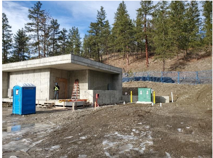
New UV building under construction.
