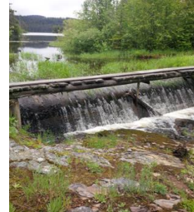
Oyama Lake Dam Spillway
