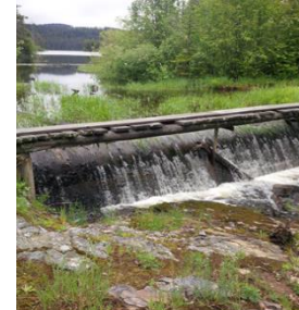
Oyama Lake Dam Spillway
