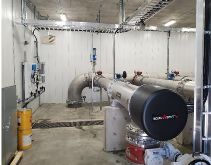
Inside New UV building
