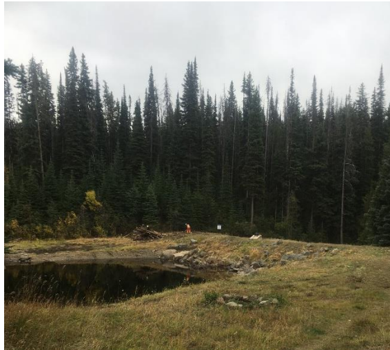
Damer Lake Dam
