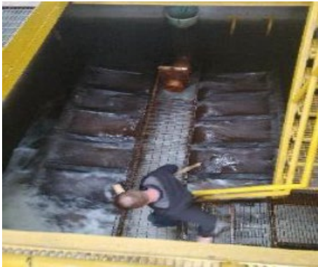
Existing Vernon Creek intake screens about to be manually cleaned
