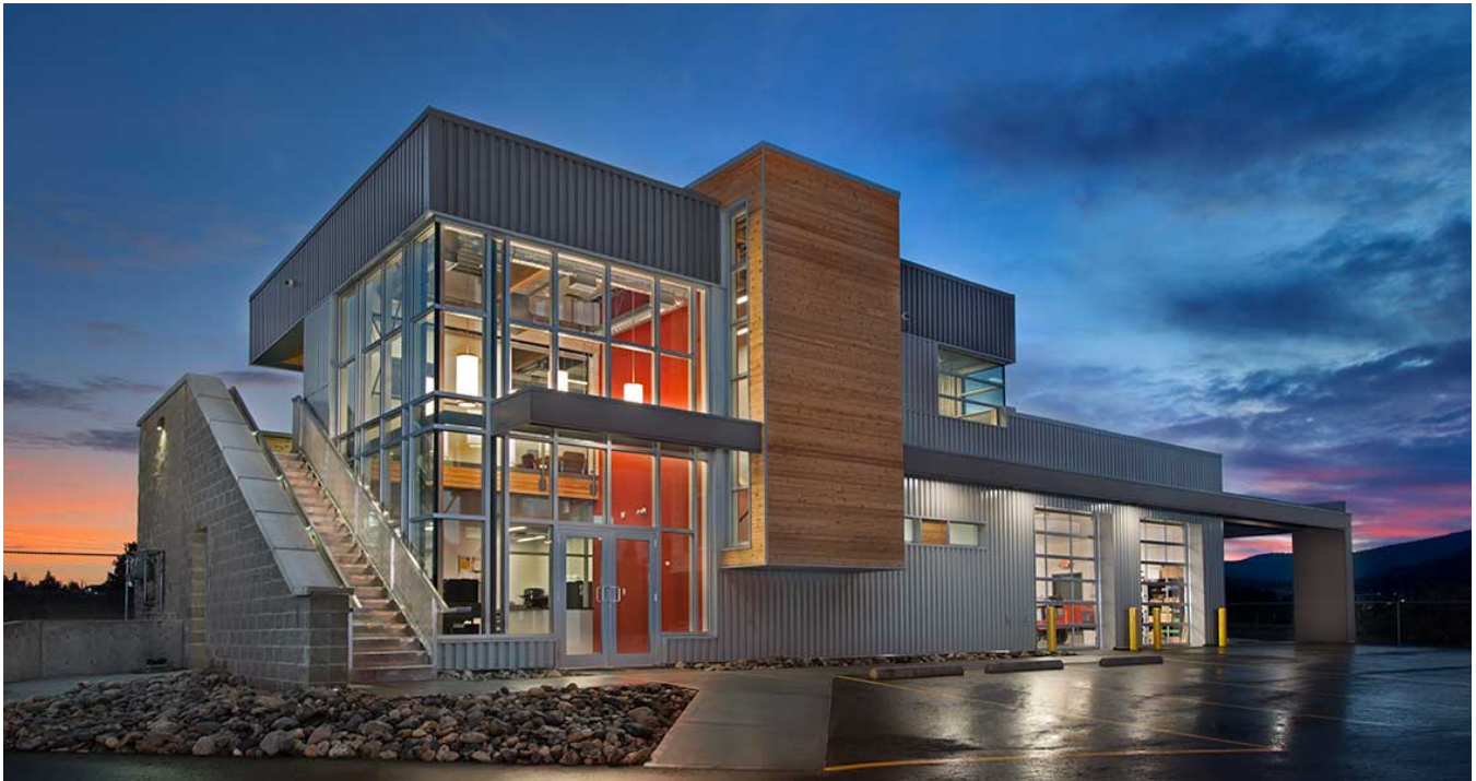
District of Lake Country Waste Water Treatment Plant
