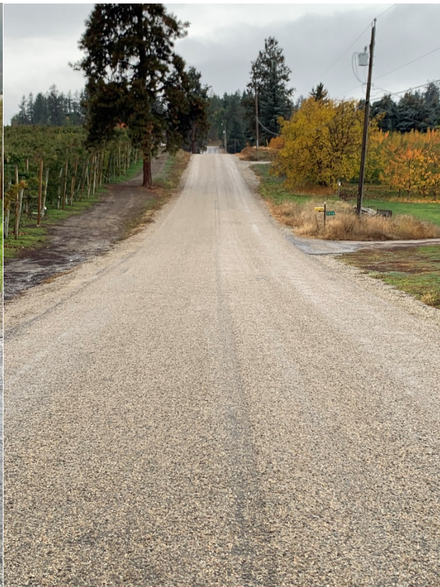
Williams Road after renewal
