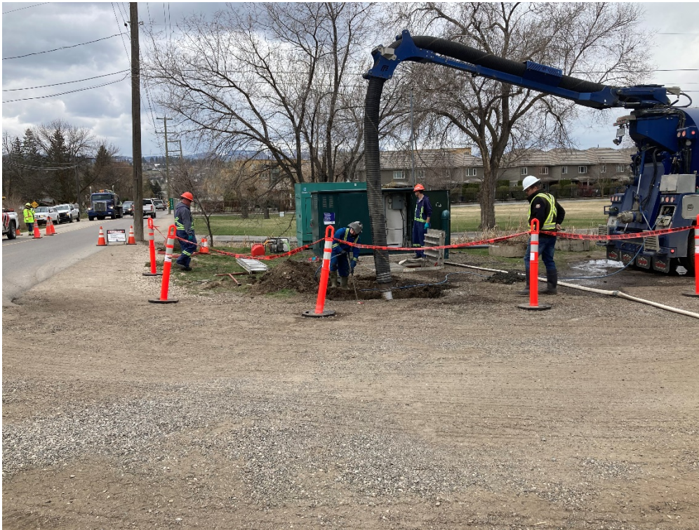
Woodsdale Lift Station - 2021 Forcemain Repair
