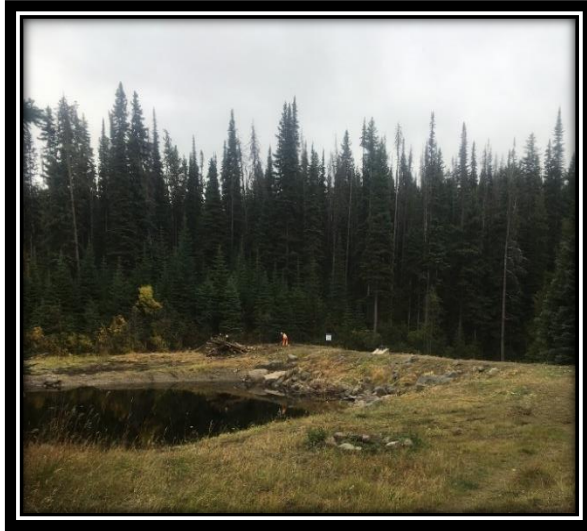
Damer Lake Dam
