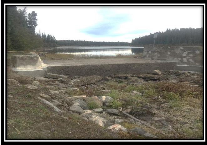
Crooked Lake Overflow Weir
