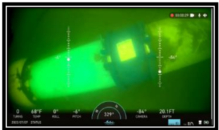
Newly installed PVC spacer spool between AC and HDPE intake pipe
