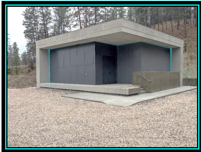
Okanagan Lake UV Facility
