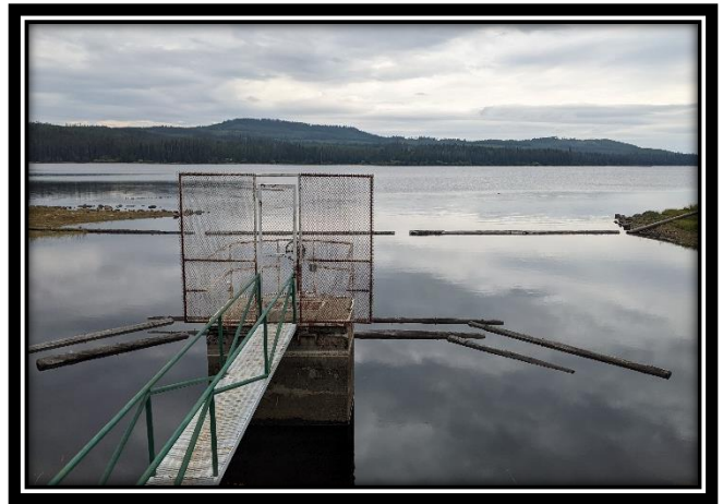
Beaver Lake Intake Structure
