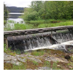
Oyama Lake Dam Spillway
