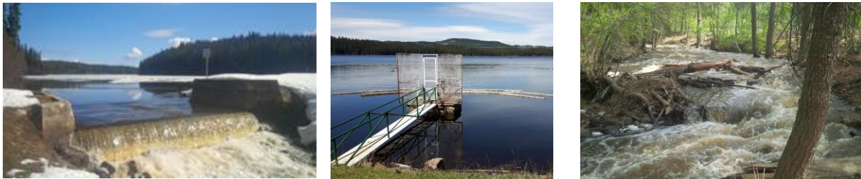
Crooked Lake (left) Beaver Lake Dam (middle) and Vernon Creek (right)
