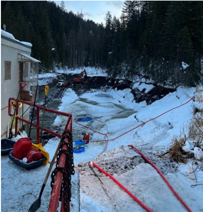
Cleaning of the Vernon Creek intake pond
