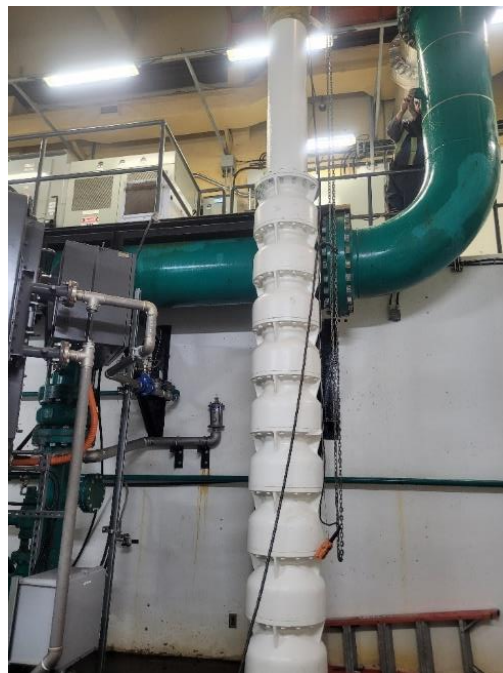
Okanagan Lake Pumphouse, lifting the pump out (left) and lowering the serviced pump back in place (right).
