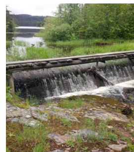
Oyama Lake Dam Spillway
