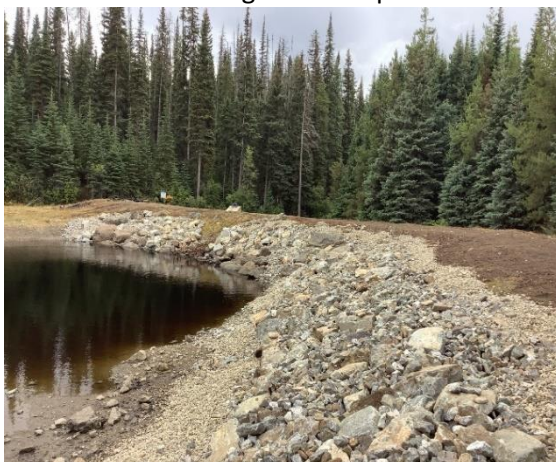
Newly placed rip rap and graded dam crest at Damer Lake
