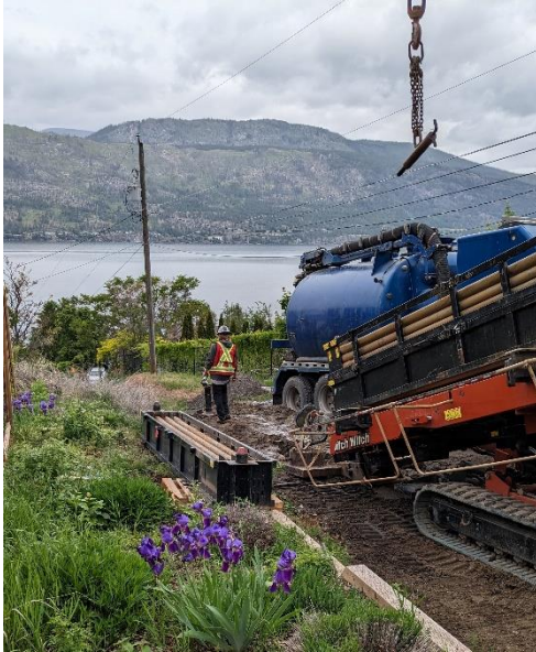
Directional drilling a portion of the new watermain (left) and the new PRV station (right).
