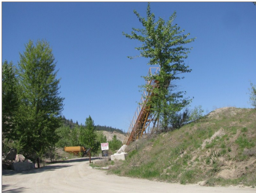
Photo 5 Entry with vegetation and berm screening
