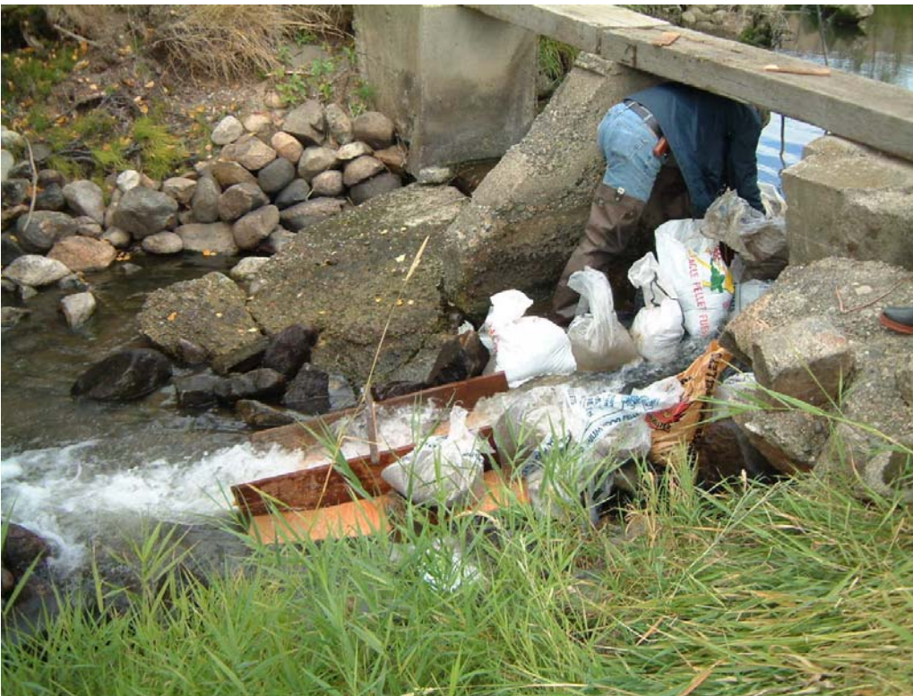
Photo 2. Fishway constructed by Ocala Fish and Game Club to facilitate passage for spawning Kokanee over irrigation dam. (Sept. 30, 2002)
