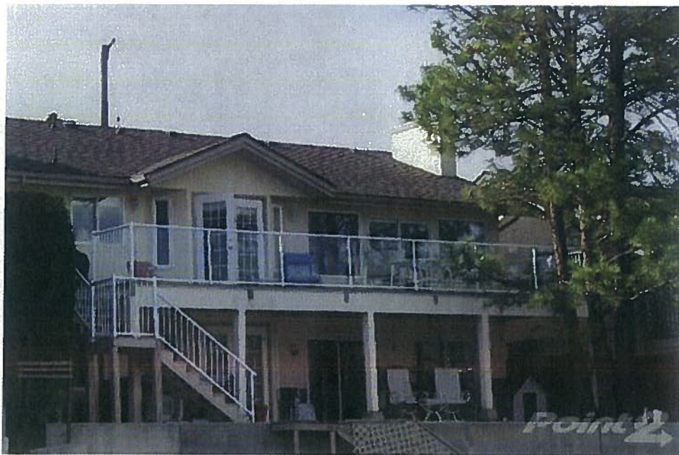
Figure 14. Example of a home with an open deck and near forest vegetation, with debris capable of igniting from ember showers.
