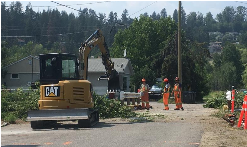
Road Crew at work
