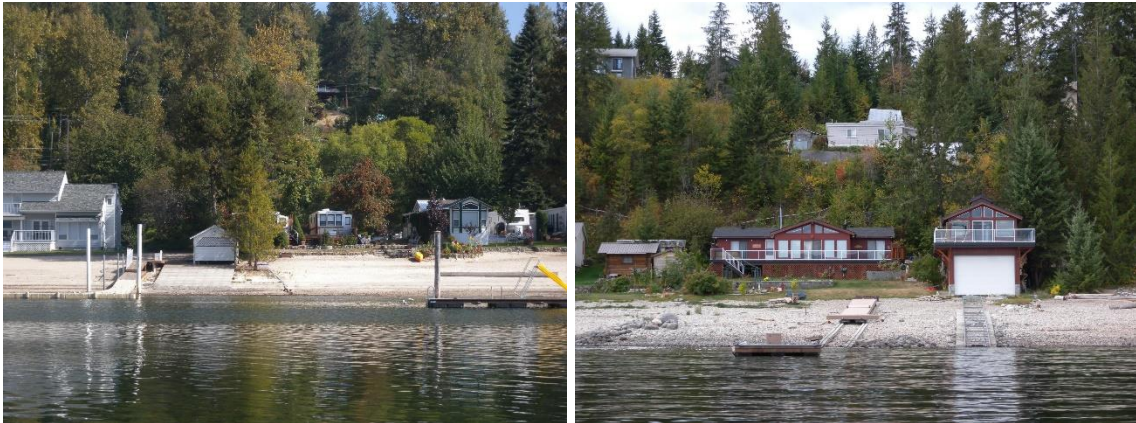
The photos above are examples of lake-access boat houses with access provided by a concrete boat ramp (left) and marine rail (right).
