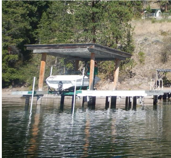
The photo above is an example of a boat cover. A pile-supported dock is also depicted in the photo.
