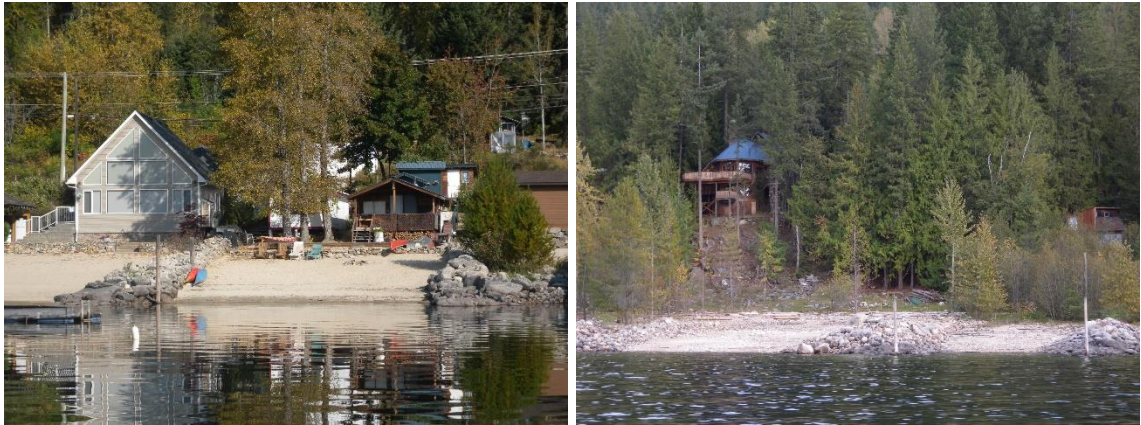
The photos above are examples of groynes constructed out of rock.
