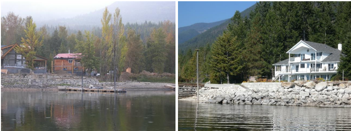
The photos above are examples of retaining walls.
