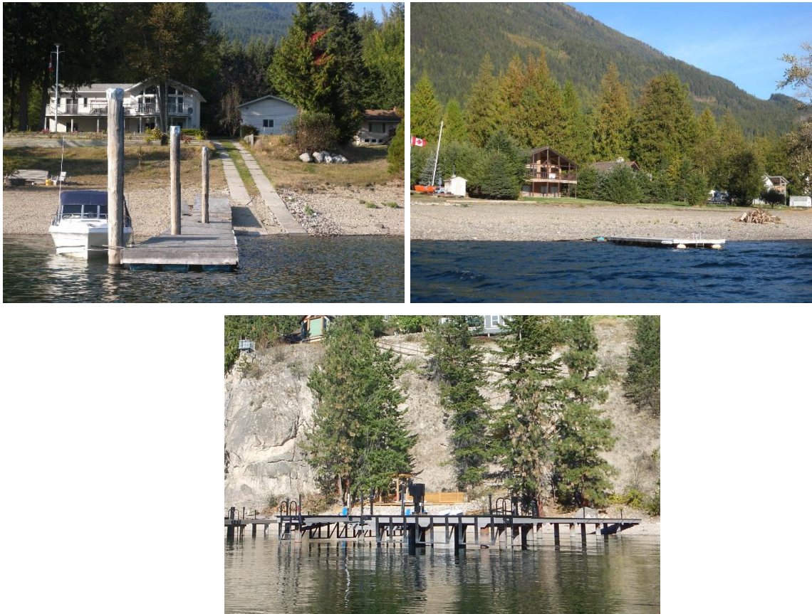
The photos above are examples of floating (top) and pile-supported docks (bottom).
