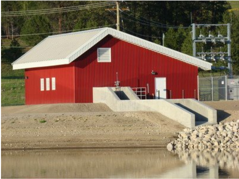
Photo 3 - Completed Generating Station from the South
