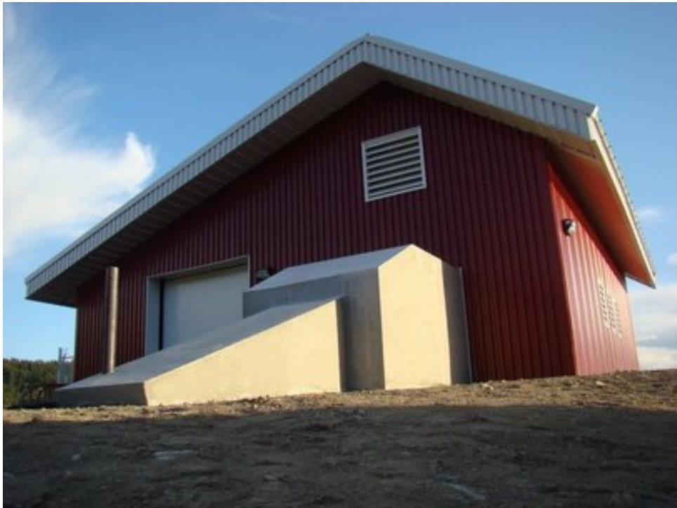
Photo 4 - Completed Generating Station from the North
