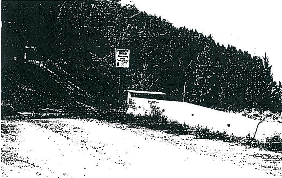
Juniper Cove Road (Single lane, with no turn around for emergency vehicles)
