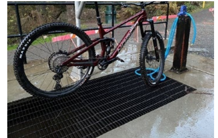
Bike Wash Station
