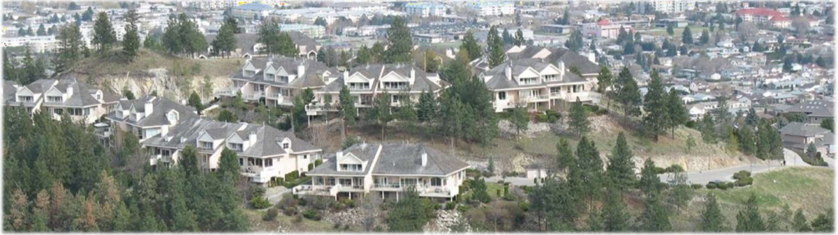
Example of Natural slope conditions maintained in yard areas, facilitating the preservation of numerous trees throughout the site.
