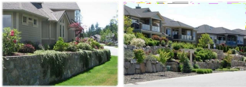
Examples of visual impact of retaining walls subdued by using context-sensitive natural materials in combination with landscaping
