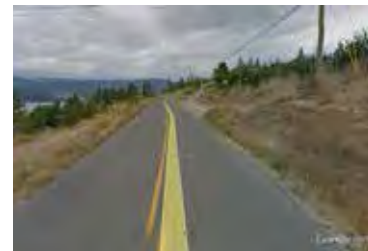
Carrs Landing Road Width: 7.2m Shoulders: 0.5m (officially 1.2m)
