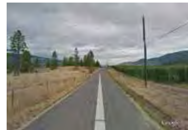
Middle Bench Road Width: 6m Shoulders: 0.5m
