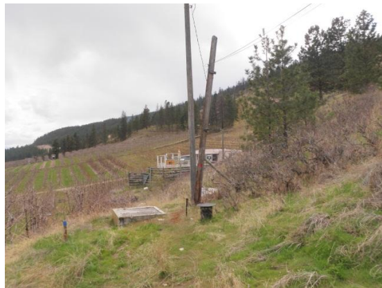
Site 1 Booster Station
