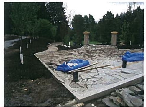
After: Main Park Entrance Under Construction
