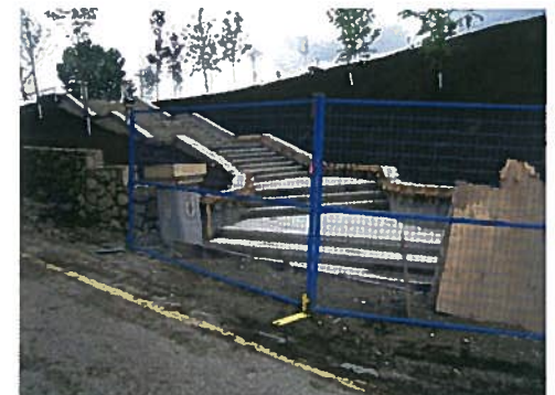
After: Grand Staircase Under Construction
