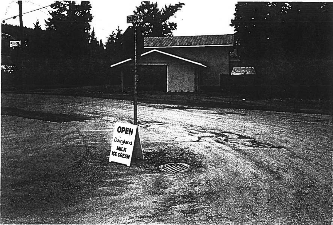
6-10 OK Centre Road West @ Fourth Street (Catchbasin)
