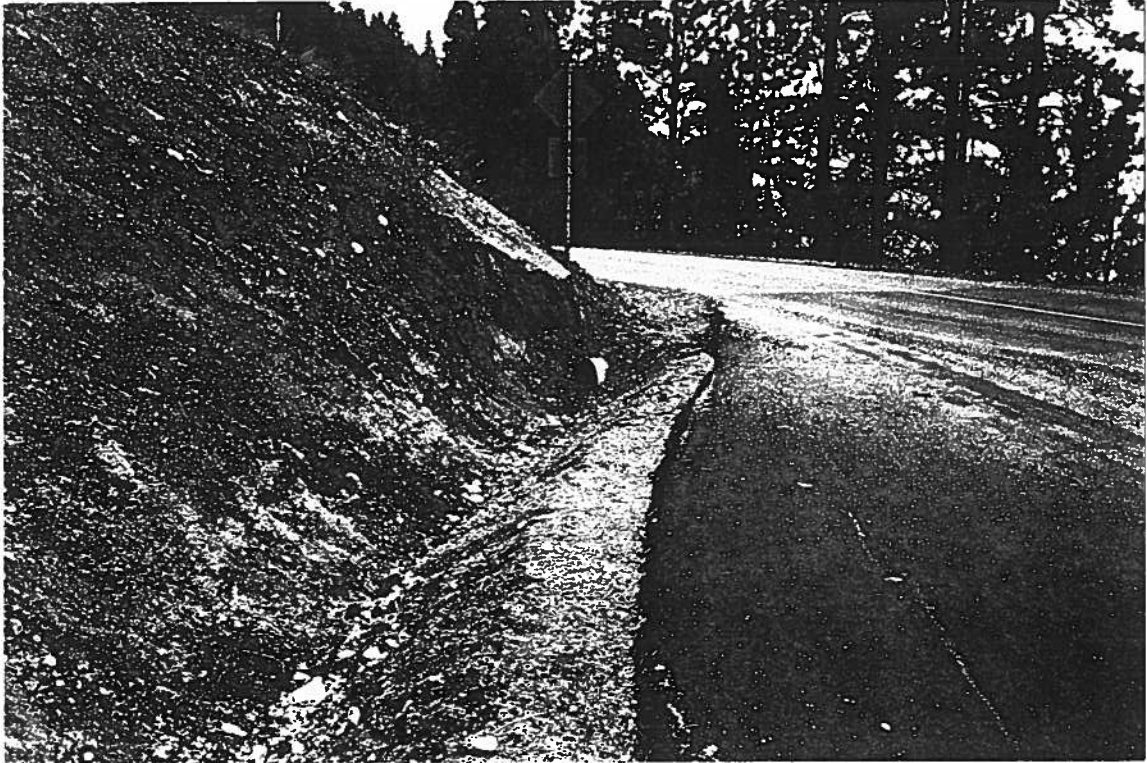
12-10 OK Centre Road West @ Fourteenth Street (Inlet)
