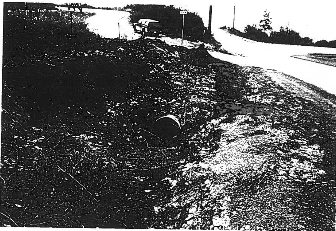
1-10 OK Centre Road East: South Ditch (Inlet)
