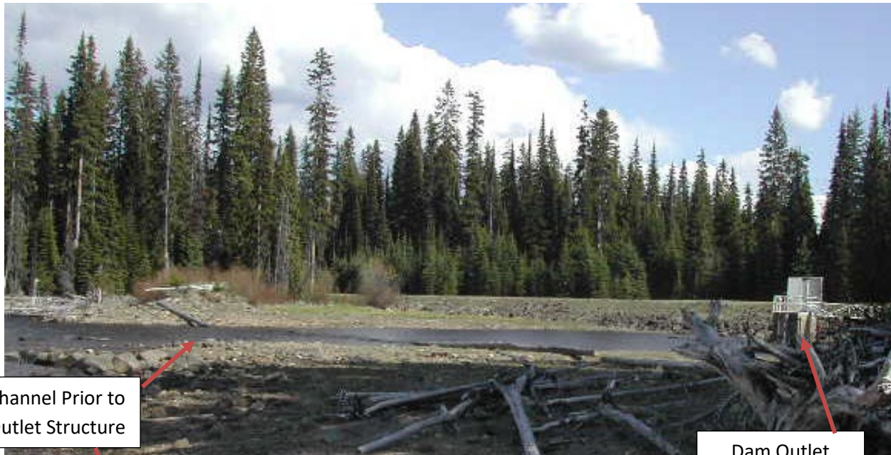
Figure 4: Channel Prior to Beaver Lake Outlet Structure
