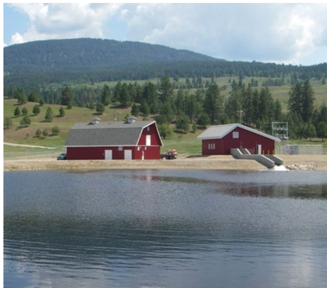
Eldorado Raw Water Balancing Reservoir
