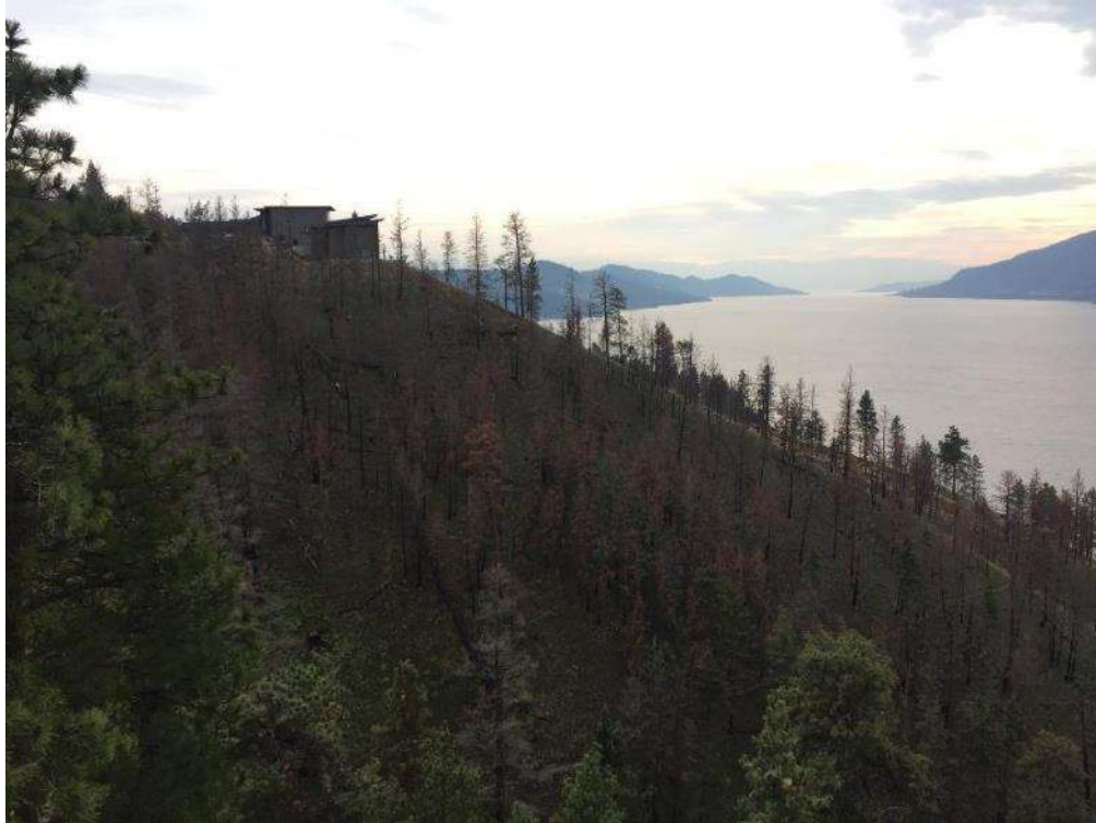
Figure 19 Structure set back in relation to the steep slope below Nighthawk Road.
